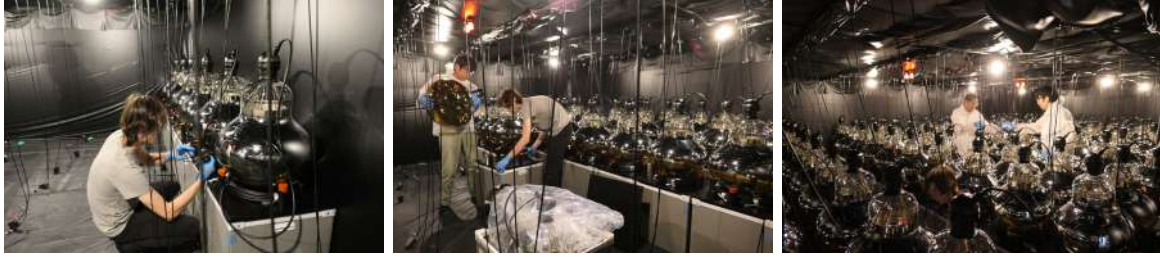
Figure 2.3: Installation work in the new dark room in Kamioka.
